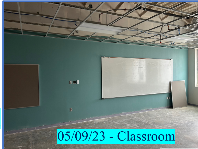
05/09/23–Wall Tile w/ Tack Strip
